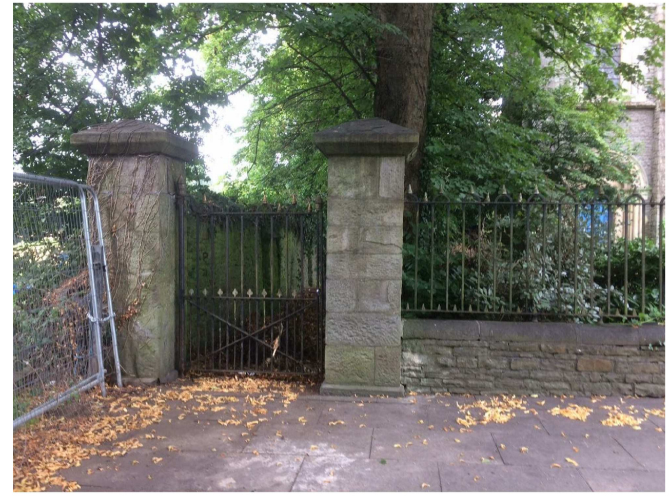
Existing Grade II Listed stone wall, gate and railings
