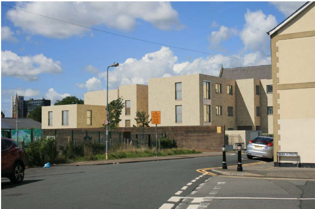
View looking north from Metal Street
