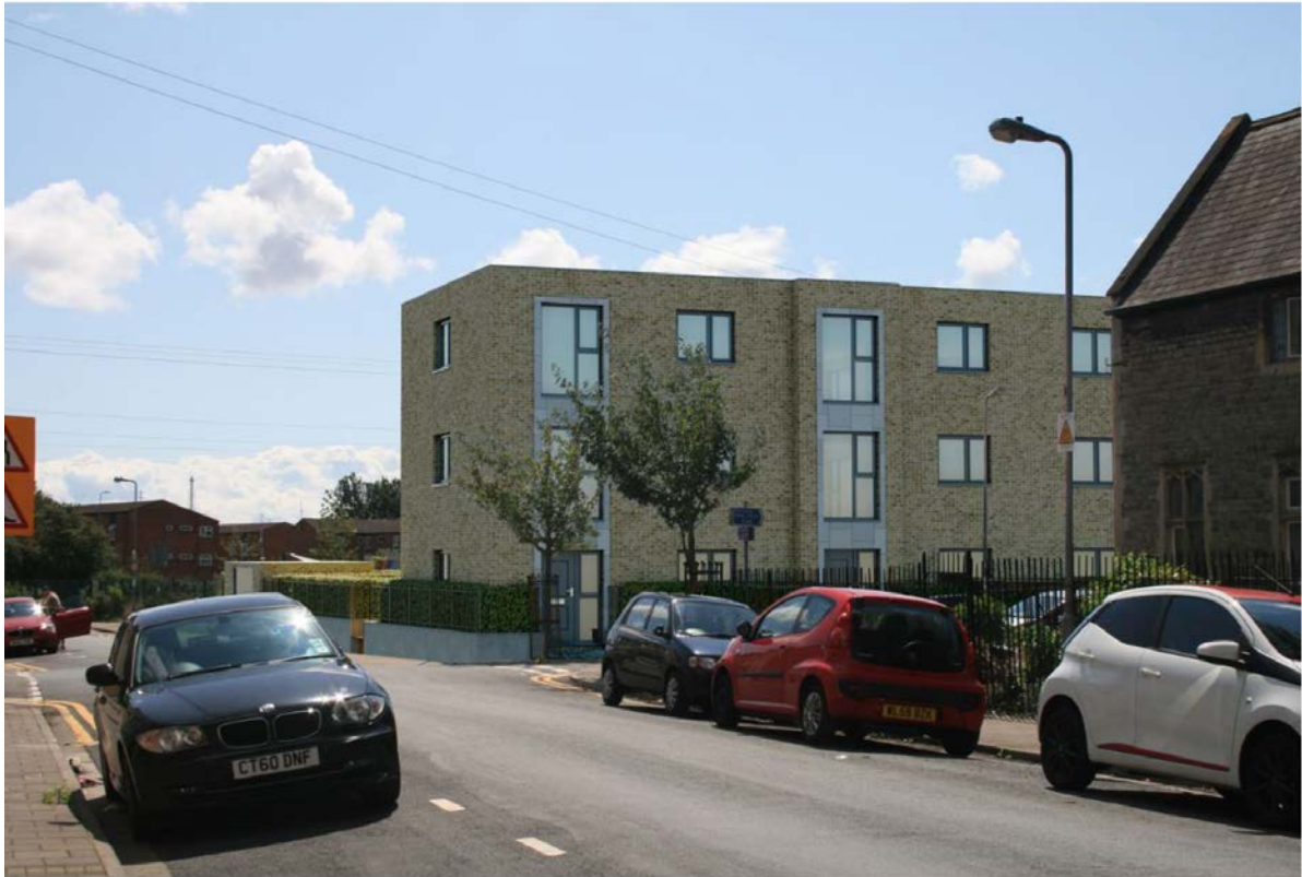
View looking south from Sun Street
